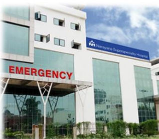
behind the hospital
